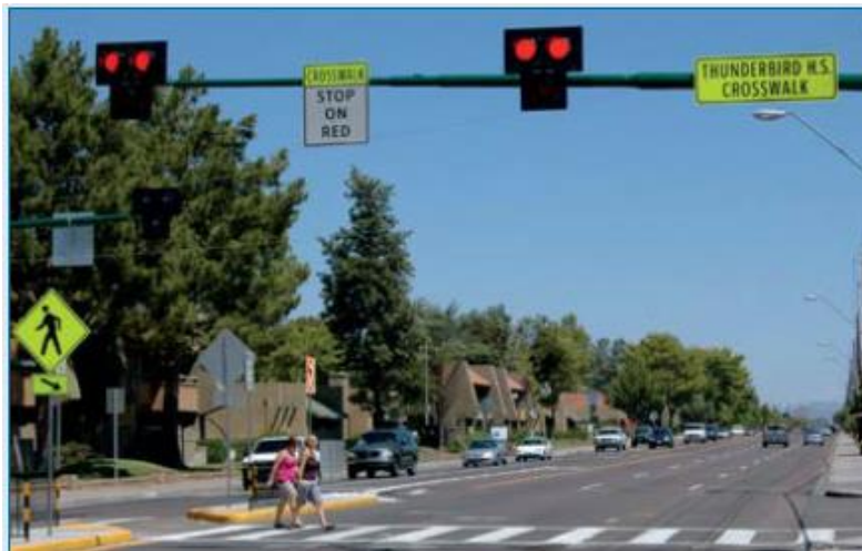
Figure 1. A PHB in Phoenix, Arizona provides protection for pedestrians near a high school.
