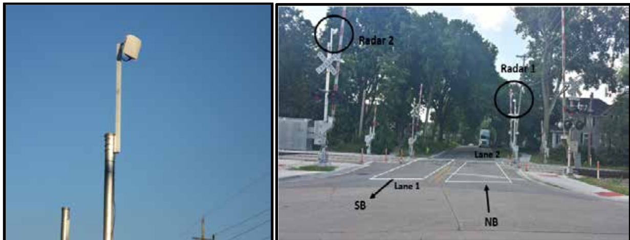
Figure 3. Detail and numbering of microwave radar units and traveled lanes.
