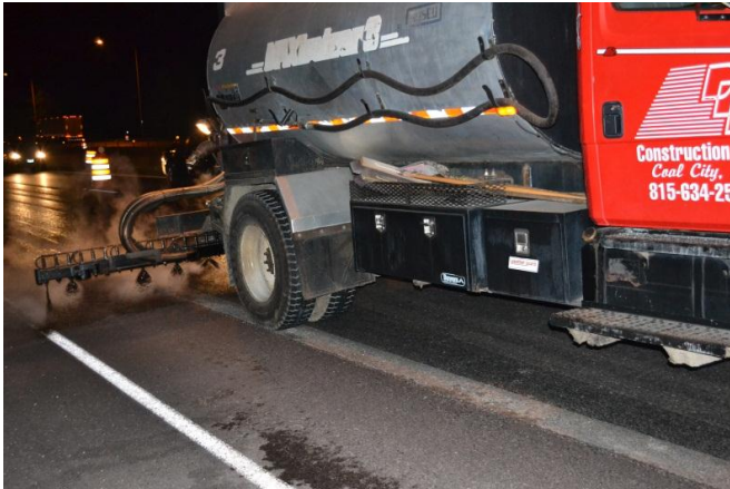
Figure 3.6. Tack coat application with distributor truck.
