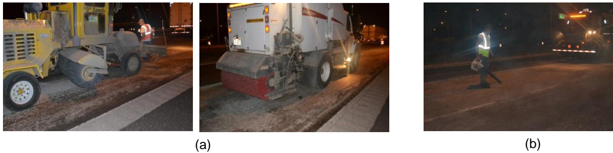
Figure 5.1. Cleaning methods: (a) Broom and vacuum, (b) Air blast.
