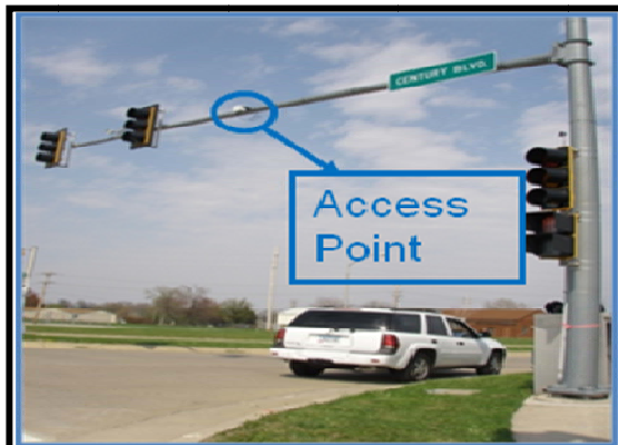
B - Detail access point.
