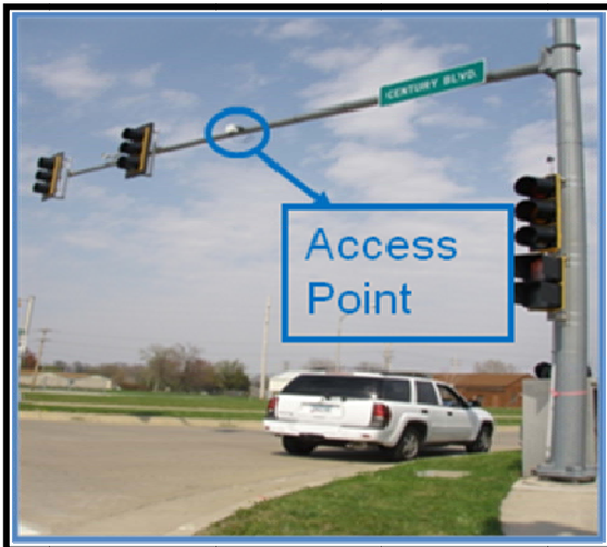
B - Detail access point.
