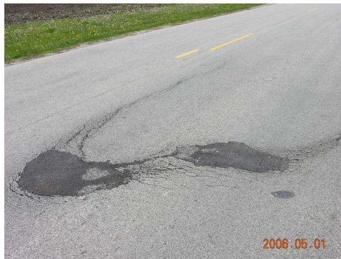
Figure 1-1. Slippage cracking caused by poor interface bonding.
