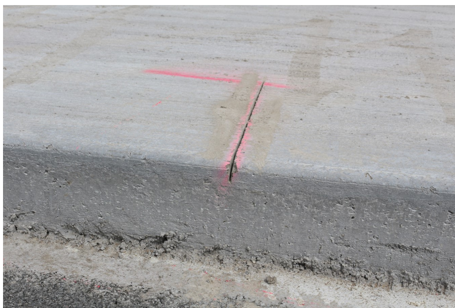
Figure 3. Photo. Active crack control saw cut notch.
