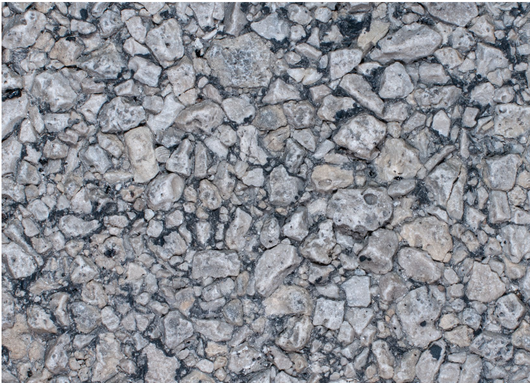
Figure 27. Photo. Overhead image acquired for newly constructed chip seal.
